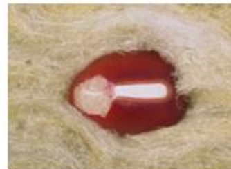
Insufficiently embedded (The cut is not in contact with rock wool.)
