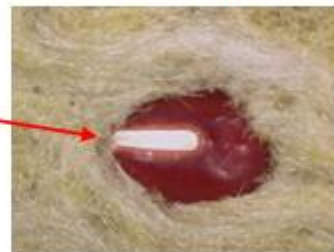
Properly embedded (The cut is in contact with rock wool.)
